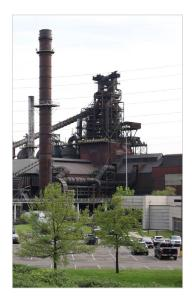
Dearborn Works relies on a centuries-old technology for crude iron production from mined iron ore: the blast furnace (Figure 2). The crude iron output of Dearborn's sole blast furnace is then refined into crude steel in either of two basic oxygen furnaces. Next, the hot, liquid crude steel is tailored into specialty steel compositions in two ladle metallurgy furnaces, before passing to a set of slab casters. See <u>GET THE FACTS: How is steel made?</u>
